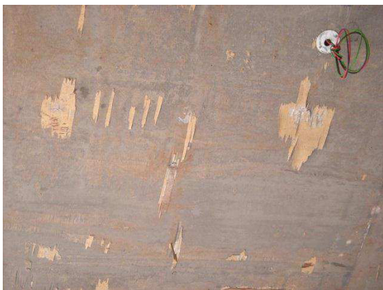
Picture 5: Plywood residual is clearly seen from the final concrete surface that used normal quality plywood as compared to High-Re FormPly in Picture 4.
