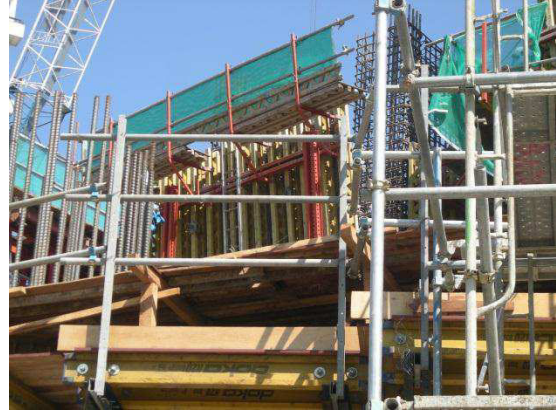
Picture 2: High-Re FormPly used in conjunction with other formwork system i.e: PERI Formwork.
