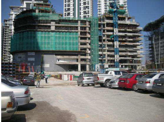
Picture 1: Platinum Park Phase 3 (Naza Tower) construction site.
