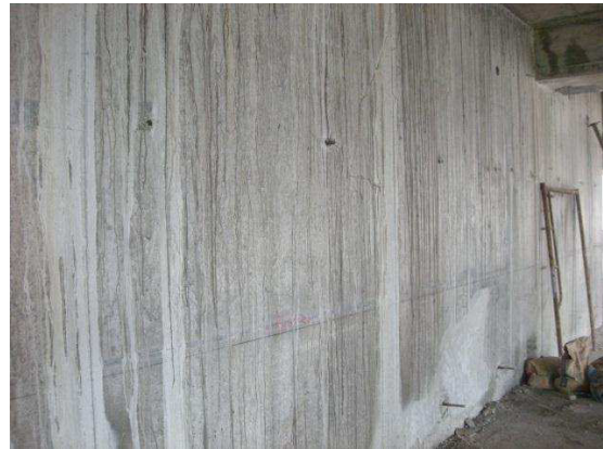
Picture 4: Final concrete surface using High-Re FormPly indicates smooth surface with minimal finishing required.
