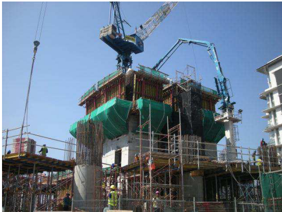
Picture 3: High-Re FormPly is used in building lift core for Tabung Haji Tower.
